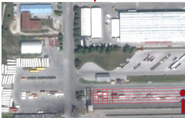
Storage position 35 D 2 in depot
